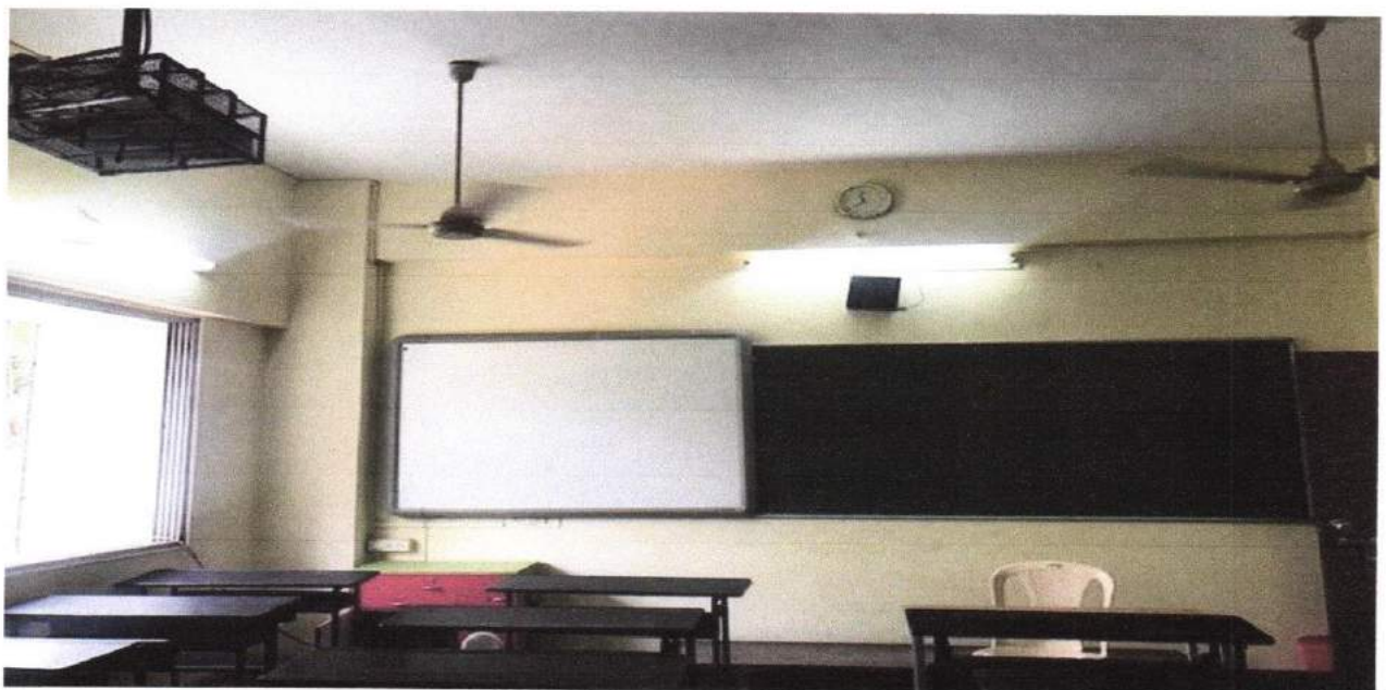
6. THIRD FLOOR ROOM NO. 45
